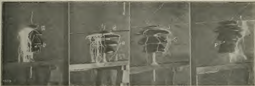
FIG. 3. FLASHOVER ON OLDEN TYPE INSULATOR.
